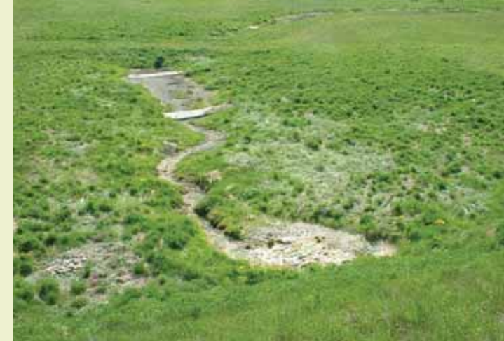
View of the Wetland from the MGEC ash settling pond
